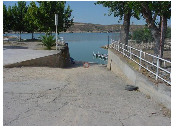
Figure 5. Reservoir access ramp with a control chain
