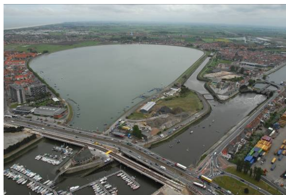
Figure 5. Aerial view of the Sluice Dock at Oostende. Photo courtesy of MUMM
